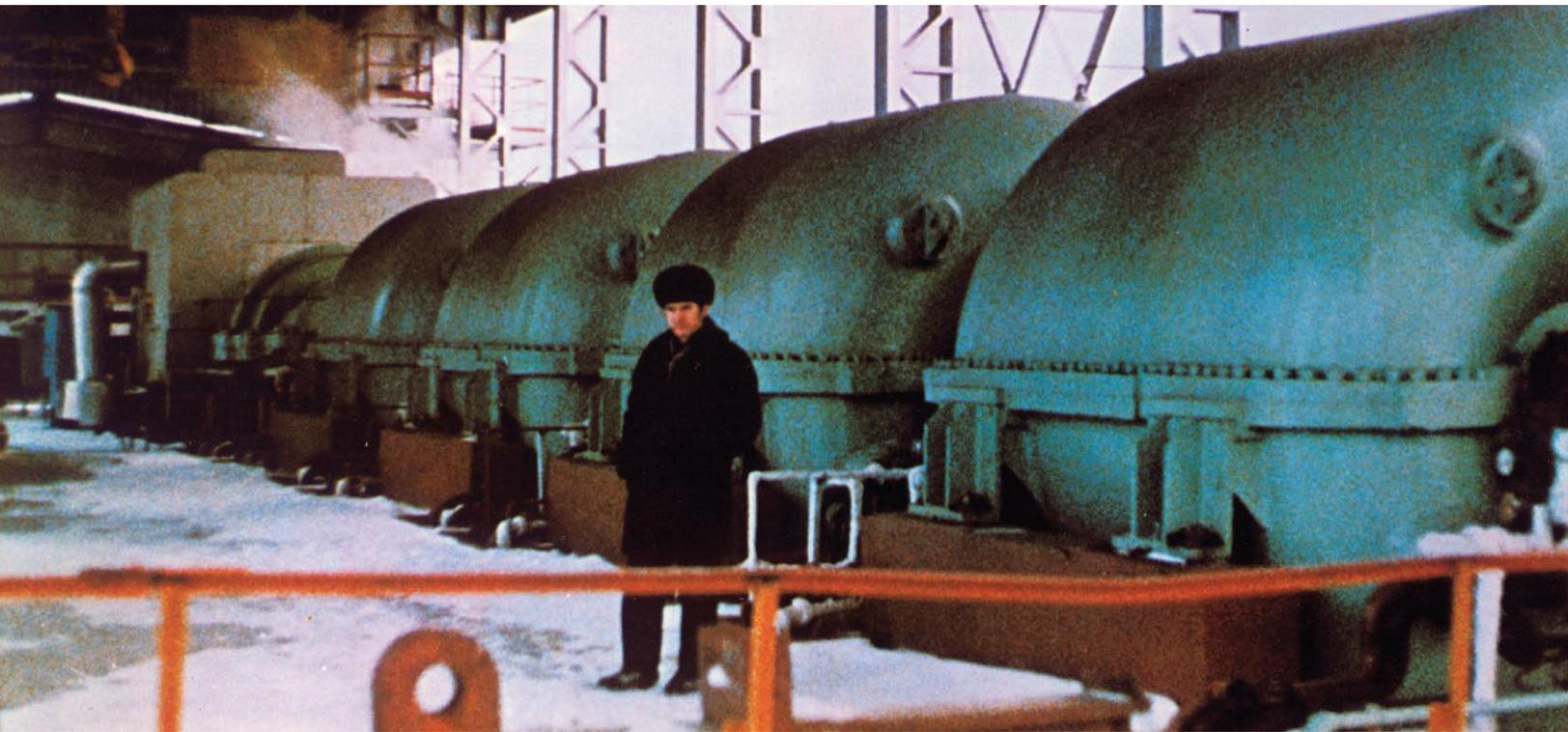
As a division of Carrier Corporation, Elliott Company became a leading supplier of gas compressors for ethylene, liquefied natural gas (LNG), refining and many other process industries. More than half of these machines were installed outside of the United States, including the compressor string pictured here in a Russian butadiene plant. During the 1970s, Elliott equipment was manufactured in Brazil, Canada, Japan, the United Kingdom, and Jeannette, Pennsylvania.
